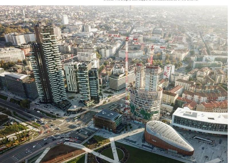
cladding, composed of double-H beams made of welded sheet metal and bolted together, on which the windows of the external "frame" will be placed. Between the central core and the external steel structure, there will be the "great void", within which a vertical garden will be created, and it will end at the top with a greenhouse.
